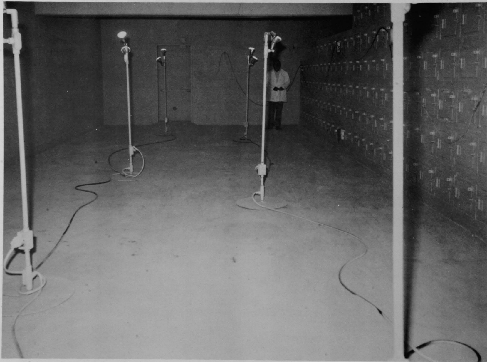
FIGURE 16. Yellow Paint Base Coat for Possible Contamination Warning in 303-C Building
